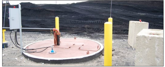
The Coal yard with the lift station
