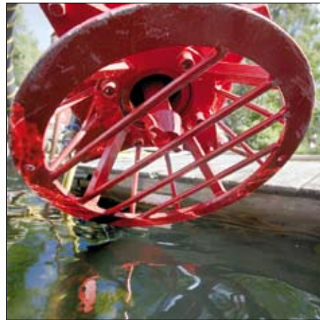
The agitator suspends solids to eliminate accumulation on sump floor.
